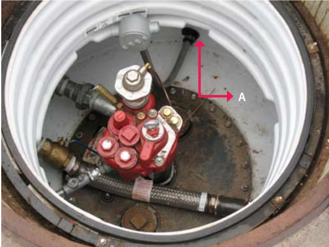
Photo 8: Contained tank sump showing the submersible pump. Rubber boots (A) seal the sump at all penetration points. These are susceptible to cracking and tearing.
