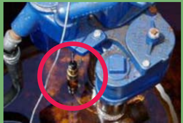
Photo 6: Examples of sump sensors.
