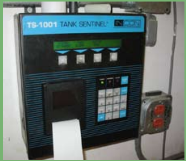
Photo 1: Examples of Automatic Tank Gauges (ATGs).
