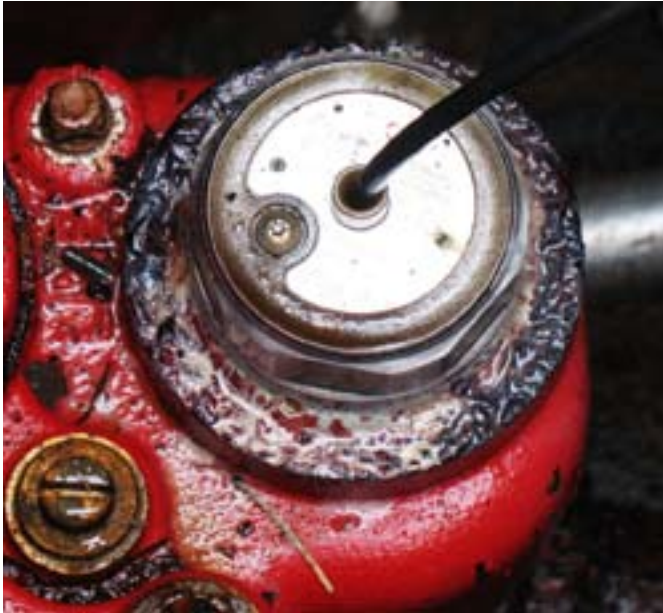
Photo 5: Example of an electronic line leak detector (ELLD).
