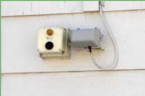
Photo 11: Examples of overfill alarms. Some alarms only come with horns (left) and some also feature warning lights (right).
