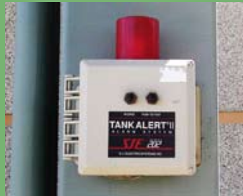
Photo 11: Examples of overfill alarms. Some alarms only come with horns (left) and some also feature warning lights (right).
