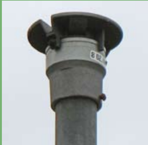
Photo 14b: Close up of the pressure vacuum vent covers.
