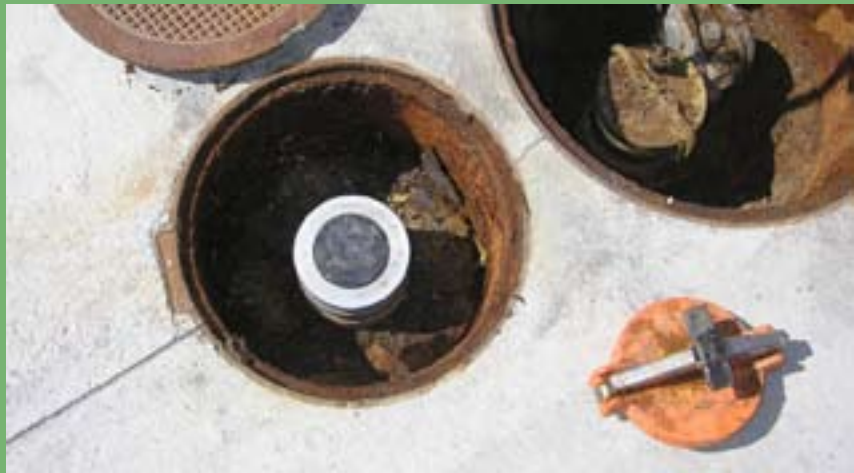
Photo 13: Dual point vapor recovery. Vapors are recovered from the riser on the left. A probe cover sump is on the right. A ballfloat is the overfill protection.
